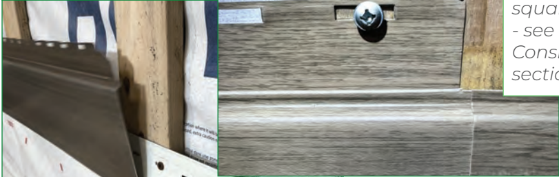
Figure 2- Hooking Aluzion Base Profile and applying even vertical pressure to set panel evenly into the starter strip.
