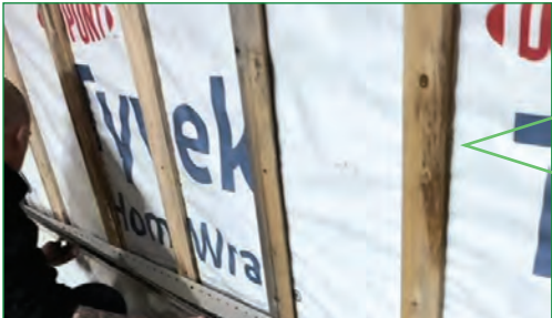
Figure 1- Hooking Aluzion Base Profile into Vented Starter Strip
