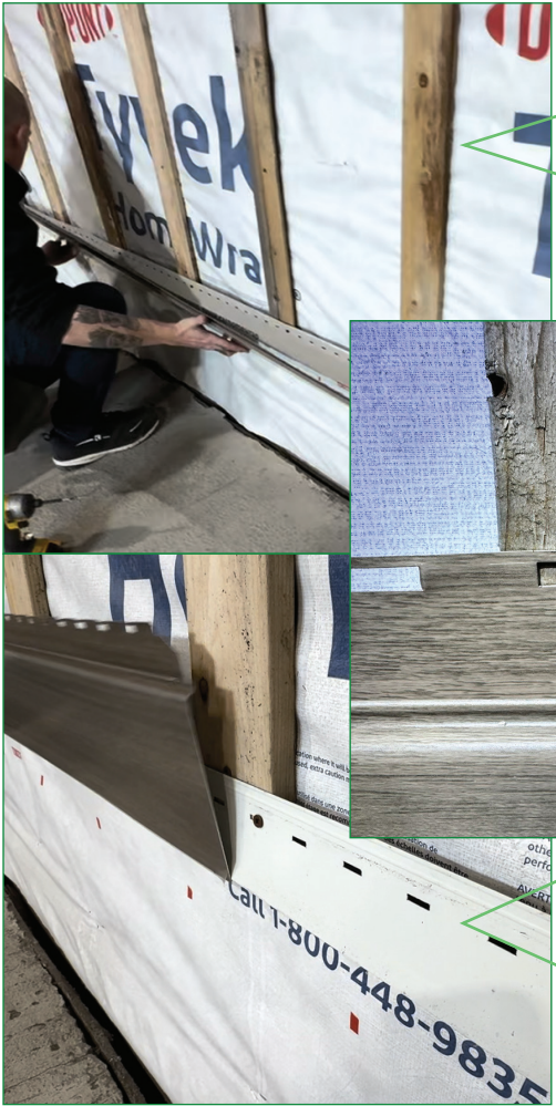
Figure 1- Hooking Aluzion Base Profile into Vented Starter Strip
